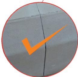
Figure 1 - Butt joint
