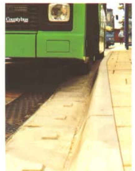
Kerbs at a bus stop in England
