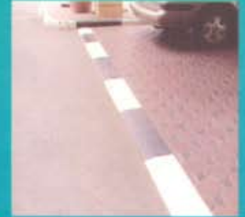
Kerbs laid flat for vehicle parking
