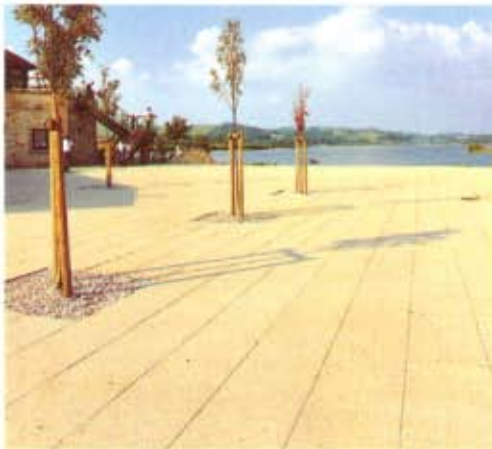
Shot blasted flags used in Sweden
