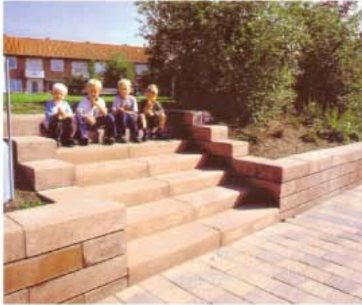
Kerbs laid flat as steps in Sweden
