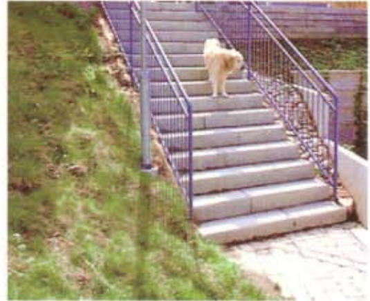
Kerbs laid flat as steps in Denmark
