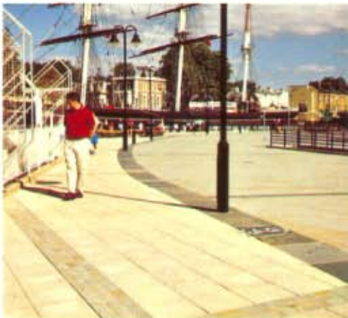
Pimple faced flags used in Denmark
